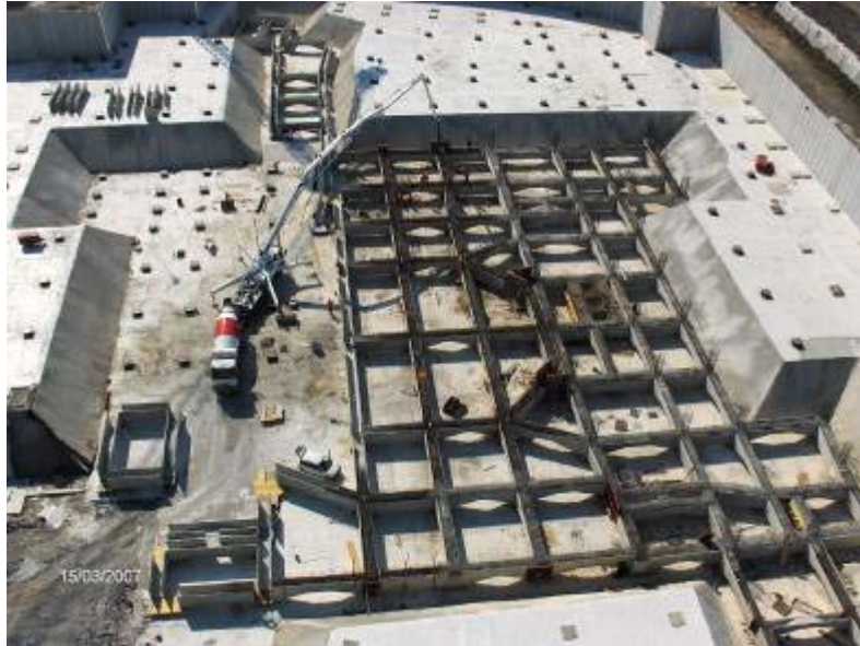
Figure 6 General view of the headquarters
