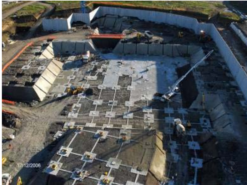
Figure 2 – View of the foundation frame on which the isolation devices have to be placed
