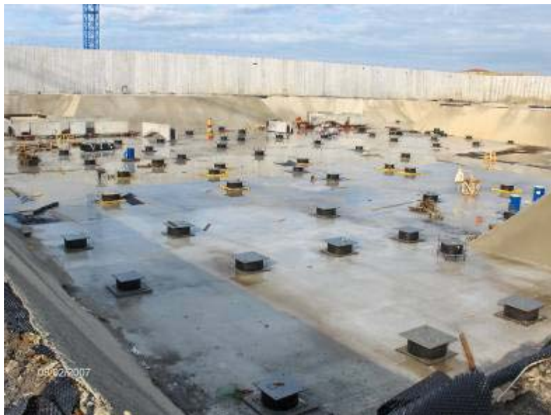
Figure 2 – View of the foundation frame on which the isolation devices have to be placed
